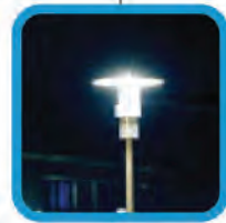
EXISTING FIXTURES EXTENDED
