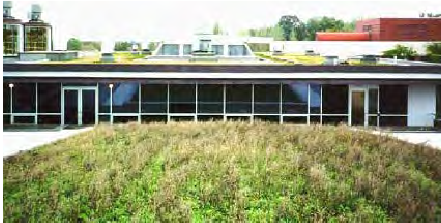
Visible Rooftop Rainwater Collection
