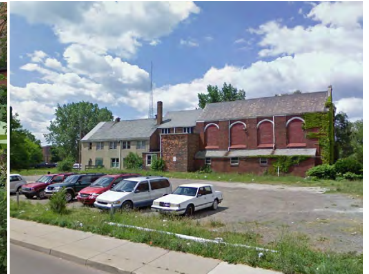
Existing church/Future culture center
