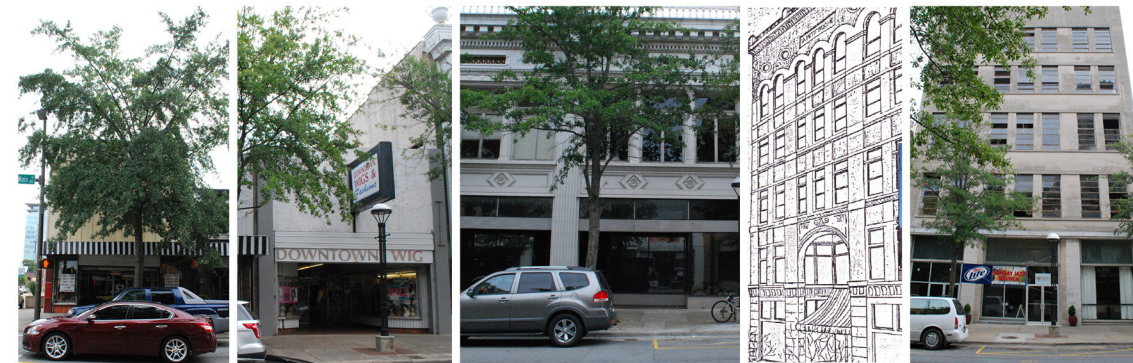
301 Main Street: Menke Building
